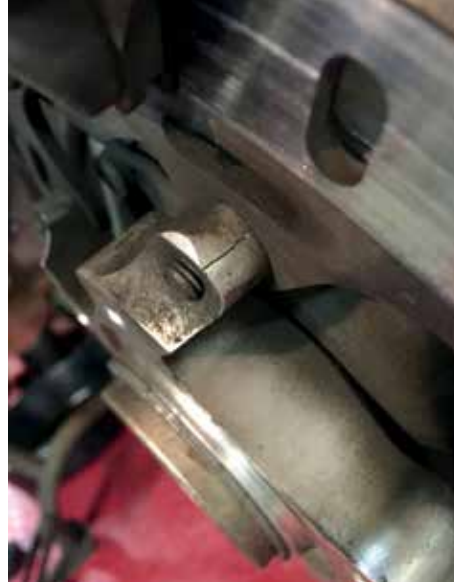
Visible flange crack.
